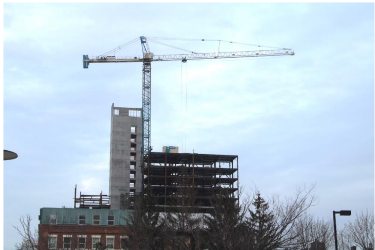
Construction in progress – The Huntington News
